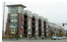
Fig. 4-23. While the cornice line, other than the dramatic corner cornice, is subdued, the color and material change of the top floor is an effective treatment that reduces the perceived scale of the building.
